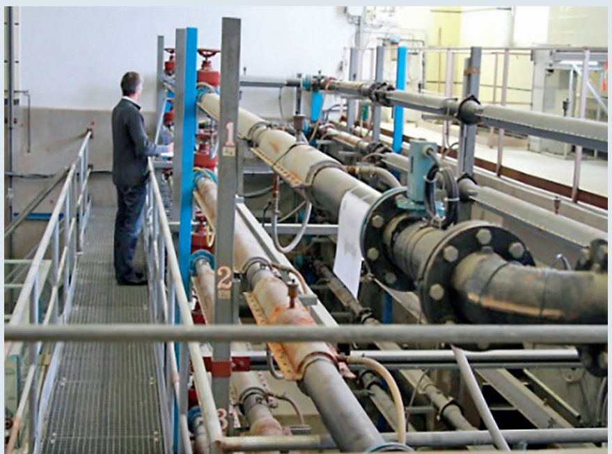
Figure 3: Use of PAMAS WaterViewer at the water treatment plant of the city of Nancy in France
